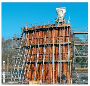
Trapezoidal Girder Formwork with steel facing
