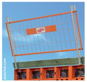
Reliable lateral protection according to safety standard EN 13374
