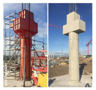
Custom formwork for construction components, where system formwork can only be utilised partially, or not at all.
