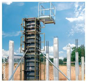
Adjustable column formwork Grip
