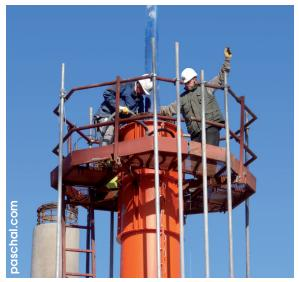
Circular column formwork Steel formwork for round and oval shaped columns.
