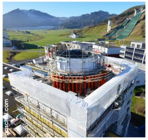
Trapezoidal Girder Formwork with plywood
