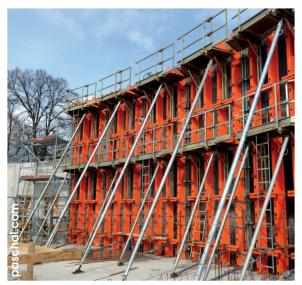
Circular Trapezoidal Girder Formwork with clamp connection
