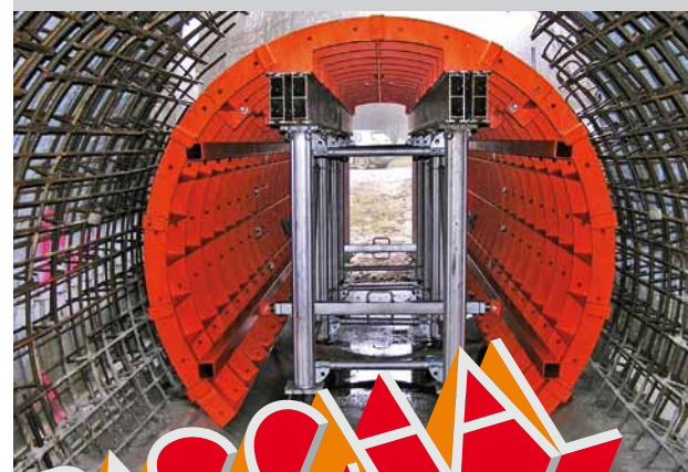
Formwork carriage – foldable formwork with GASS shoring system F-Haudiomont, Fa. Berthold s.a., F-Dieue sur Meuse
