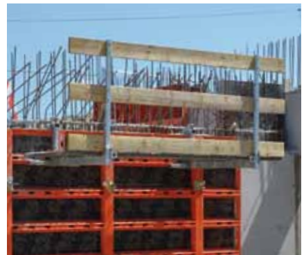
Concreting platforms can be folded for transport or storage to save space.
