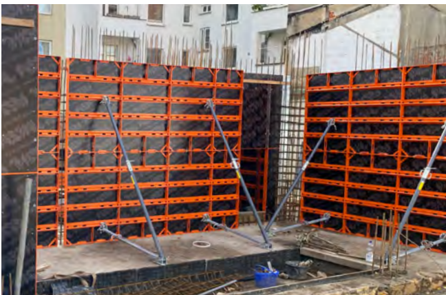
The lightweight formwork NeoR has been extensively tested and is ready for use in a wide variety of fields.
