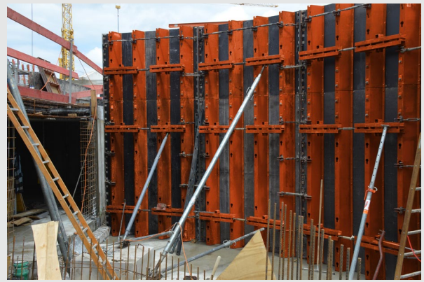
Adjustable prop 175-285 cm on a construction site in Ringsheim
