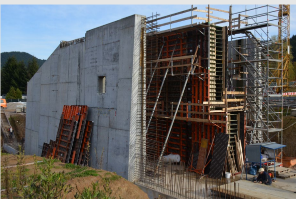
Adjustable prop 620-1000 cm on a construction site in Welschensteinach
