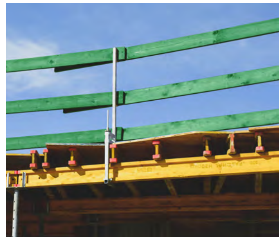
The Secuset lateral protection system can be installed safely and efficiently on the H20 wooden girders.
