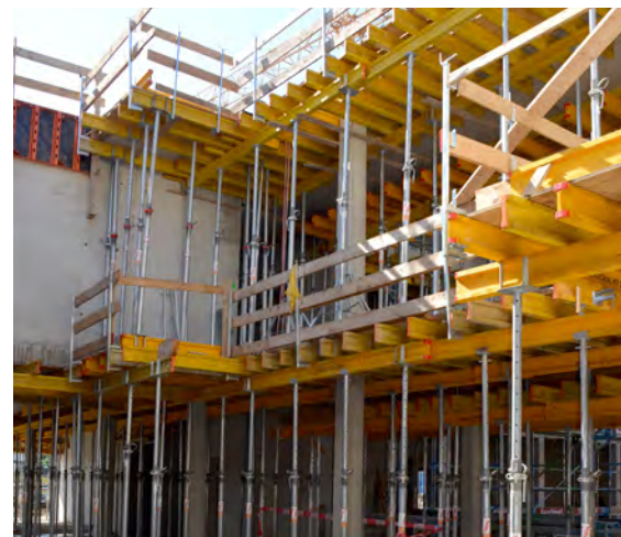
The H20 beam is overlapped in both directions in the PASCHAL Deck slab formwork as a yoke beam and cross beam and thus adapts flexibly to any room size and geometry.
