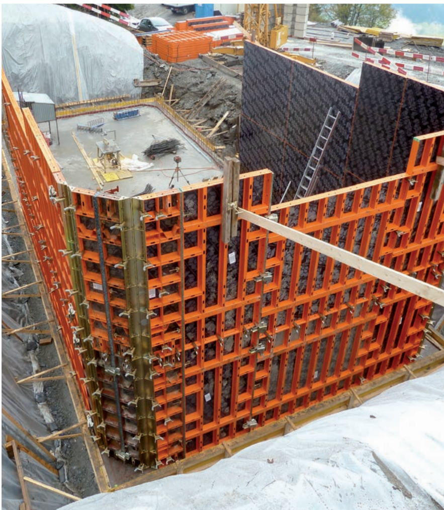
Wasserreservoir Surcuolm, CH-Obersaxen GR; Candrian SA, CH-Illanz
