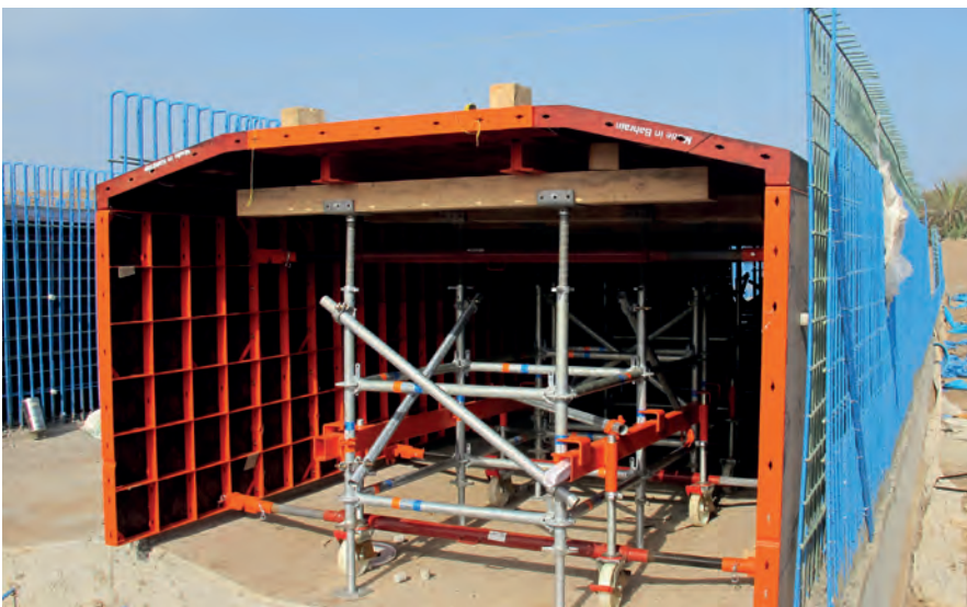
Box-Culverts, OM-Suvar ; Sté. NCC Limited, IND-Hyderabad
