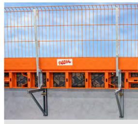
Safe working with at the slab edge combined with the Secuset lateral protection system.
